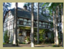
North Side (Main Entrance) of House
